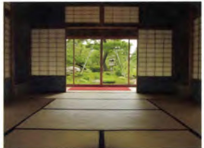
FIGURE 7-25 Teahouses are designed specifically for the tea ceremony. Sliding doors are made of wooden lattices and paper. Tatami mats, traditionally woven from rice straw, cover the floors. An ideal teahouse also has a garden for guests to enjoy. This teahouse is in Kanazawa, in western Japan.
