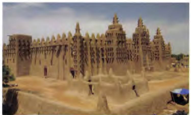
FIGURE 8-25 The Great Mosque of Djenné, in Mali, was first built as early as 1200 CE. It became an important Islamic learning centre during the Middle Ages.
