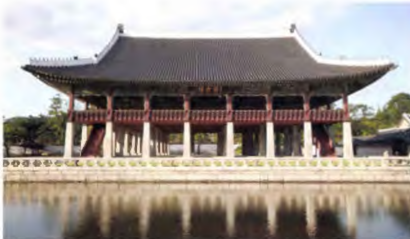
FIGURE 12-14 Wide eaves make a house cooler in the summer. This building has a single eave supported by columns. Some palaces and temples were made with multiple eaves. Why would an architect choose to do that?
