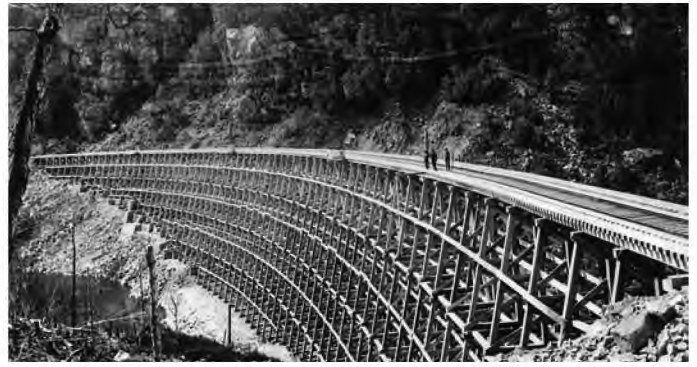
FIGURE 5-33 This wooden railway trestle, 33 m high and 270 m long, is in Ontario. Look closely at the landscape and the scale of the bridge. Even though it was the cheaper option, what kind of time and resources would have been spent to build this bridge? How many wooden bridges do you think were built across Canada?
