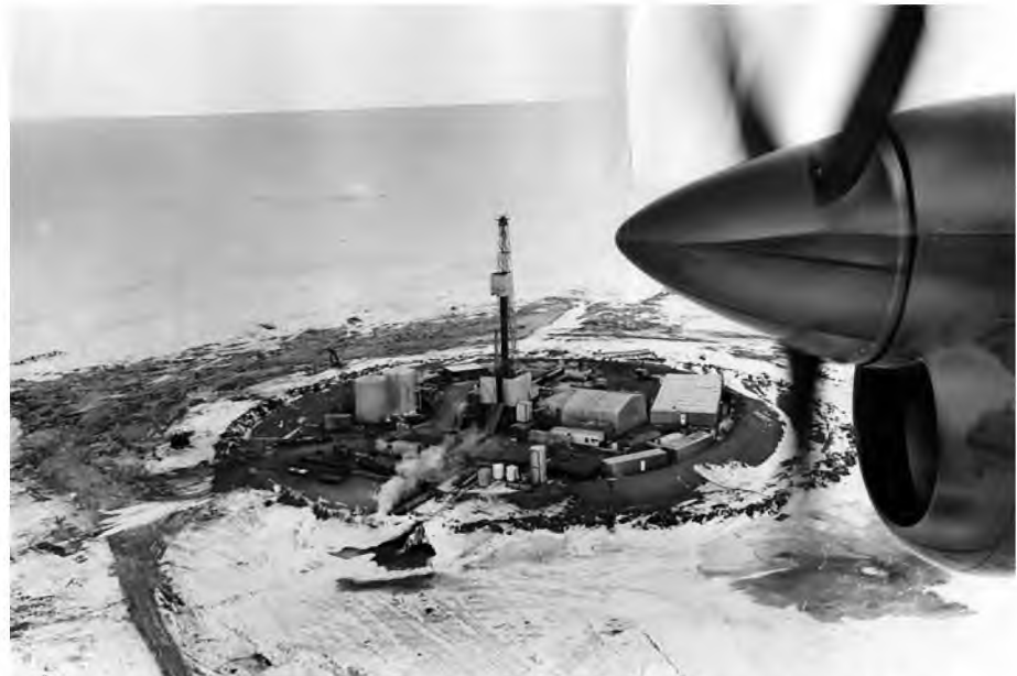
FIGURE 8–21 In the 1970s and 1980s, oil companies constructed artificial islands on the Beaufort Sea so that drilling platforms could be built. Because of permafrost and Aboriginal concerns, the construction of pipelines was delayed, and the Beaufort Sea oil reserves were left untapped. Do you think this decision might change in the future? Why or why not?
