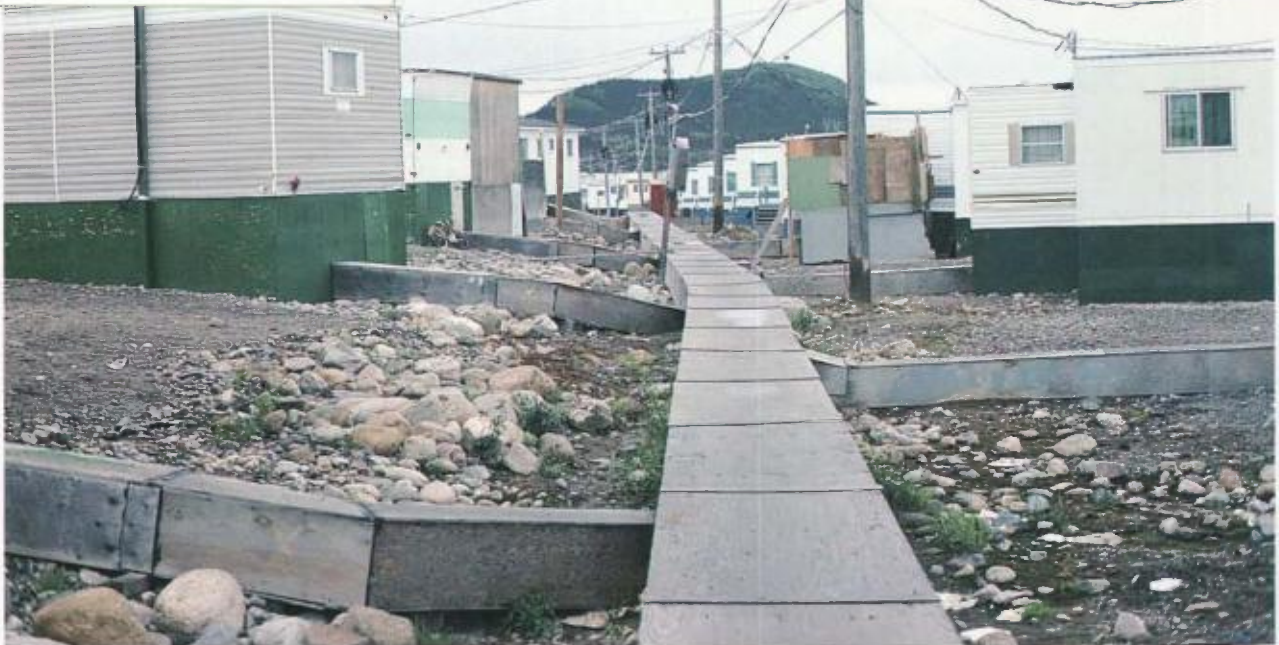
Figure 6-51 Utilidors in Iqaluit
