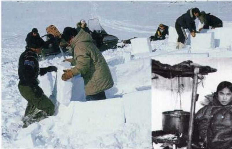
Figure 7-3 Left: Two people working quickly can build an igloo in a matter of hours. In the western Arctic, the Inuit build pit houses (an example is on page 203). Right: Inside an igloo. The women are seated on a raised platform. The cooking area is to the left.
