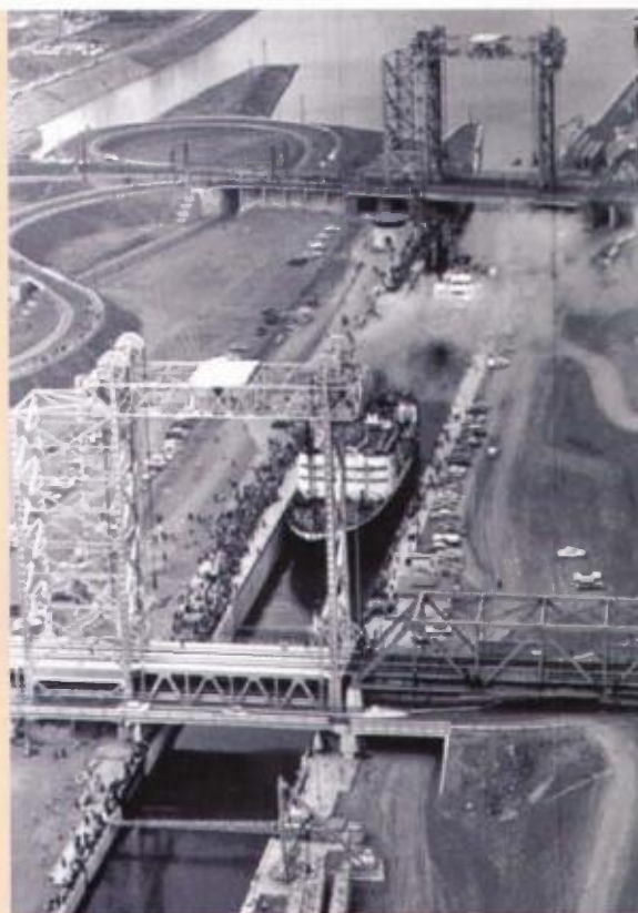
Figure 7-9 An ore carrier enters St. Lambert Lock on the St. Lawrence Seaway.
