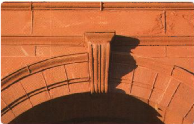
Figure 8 If the keystone of this arch is removed, the arch will collapse.
