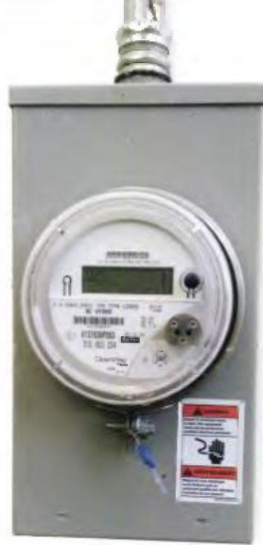
Figure 3.29 Smart meters measure electrical energy use as it changes over the course of the day.
